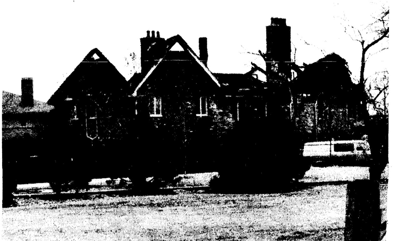
Above is what remains of a home on Elmsleigh Lane that was severely damaged by a two-alarm fire last weekend. Officials don't know what caused the blaze and estimate damage between $300,000 and $500,000.
