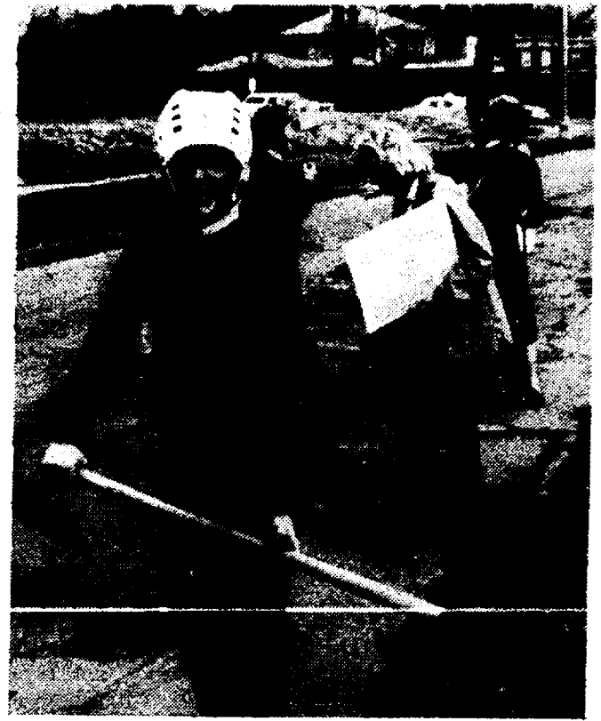
This was the scene in April, 1982, when Mothers Against Potholes donned hockey helmets for protection and began patching the crevices on Lakeshore Road to draw attention to the county road commission's refusal to maintain the street. The county said it was Grosse Pointe Farms' responsibility to pave the county-owned street. At left is Alexandra Mackey, one of the mothers. Now, Grosse Pointe Woods is continuing its fight with the road commission over another county road, Mack Avenue.
