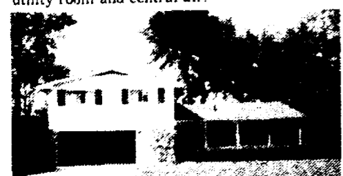
30 PUTNAM PLACE What more could you ask for than a secluded, quiet location, four bedrooms, 2 1/2 baths, first floor utility room, family room with wet bar, breakfast room & central air.
