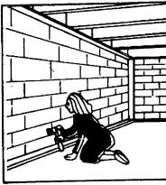
FIGURE 1 - Homeowner nails 2 x 2 bottom plates to base of wall with a ham-mer and special masonry nails.
