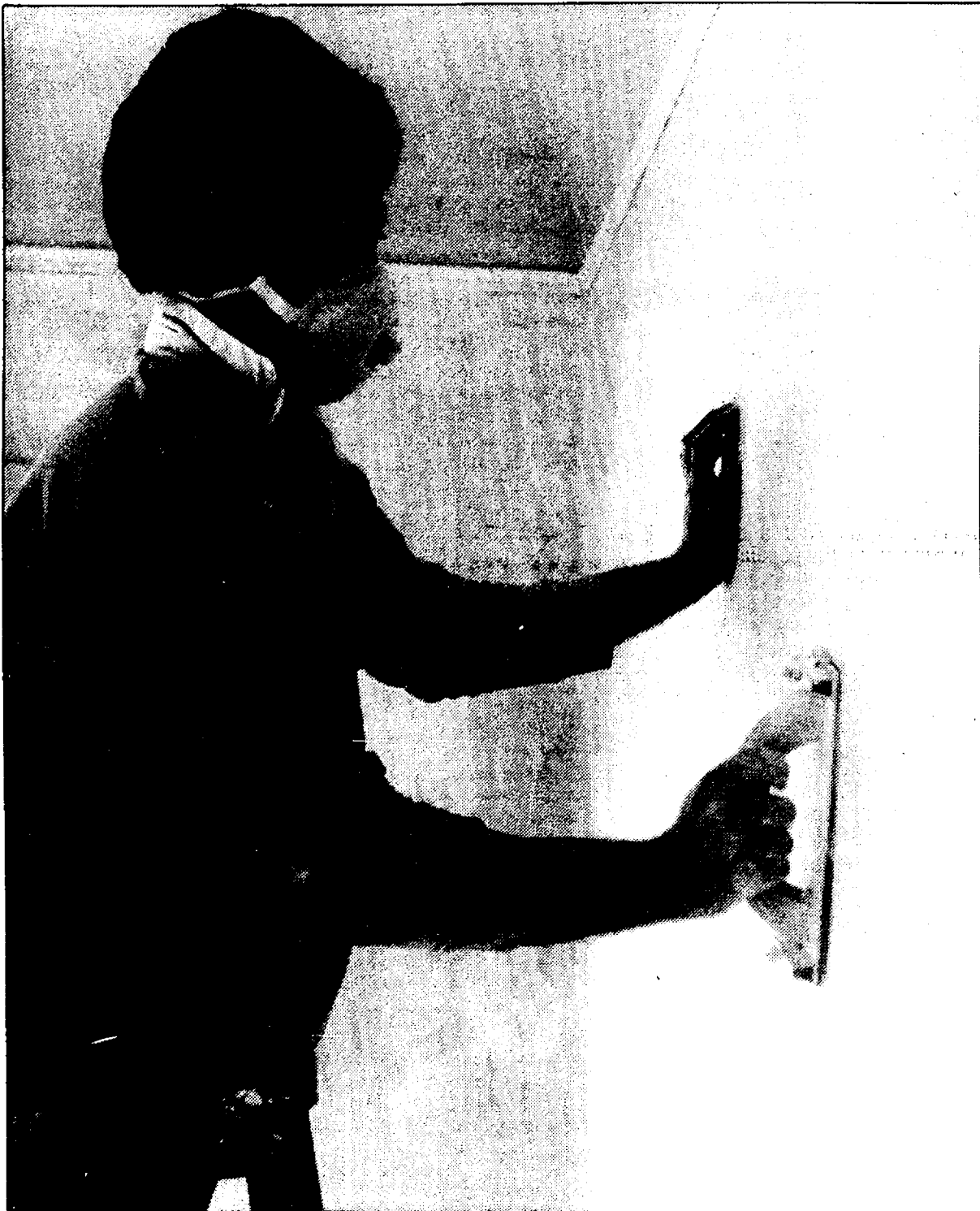
A lot of handwork went into preparing the Showhouse. Here, custom painter Michael Meda sands a wall in the master bedroom to prepare it for painting and glazing. Meda worked for five days to paint this room with a base coat and successive layers of glaze that were cross-combed for a textured effect.
