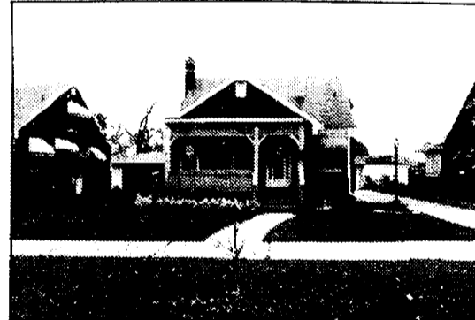
16524 TOEPFFER — East Detroit — nice location. Sharp, custom three bedroom brick bungalow with a brand new professionally built kitchen, all new porch, privacy fence, and deck in the back. Other features include a new air conditioner, two and one half car garage, and much more. $56,900.
