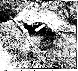
The plastic pipeline can be seen here through α hole in the existing sewer on the north side of Lakeland.
