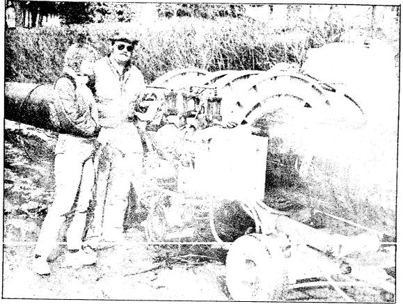
Placing piping in the existing sewers on one block of Lakeland is a tricky task. Carol Smallish, of McNamee, Porter and Seeley, looks on as John Baily of Ryerston Steel works on the plastic fusion unit. The unit connects large segments of plastic pipeline. That pipeline is then inserted into an old storm sewer line without having to dig up and replace the entire line.
