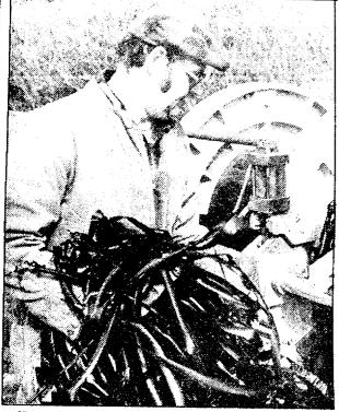
Here Baily gathers shreds of plastic that have been sheared off the thick plastic tubing to make both sides of the joint fit flush together.
