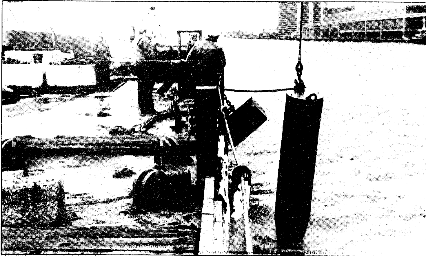
Workers must lift out the winter buoys which have become heavily scraped from winter ice and replace them with fresh buoys. Note the block in the center of the photo. That sinker probably weighs about 1,000 pounds.
