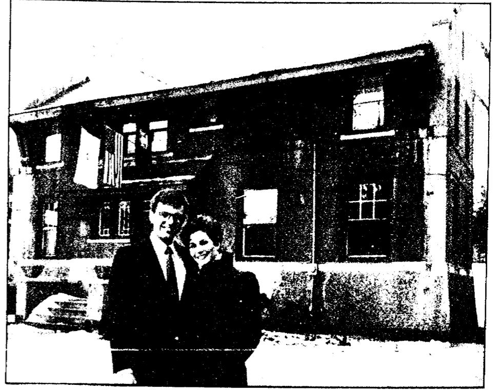
John and Julie Dyle stand before the house they're renovating. It was built more than 80 years ago as the first telephone exchange for the Grosse Pointe area. It held the switchboard and the offices for the local phone company until the late 1930s.
