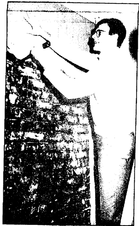
John Dyle chips away at some plaster in the living room of his 82-year-old house. The walls are three bricks thick — an old fashioned method of fireproofing a building.
