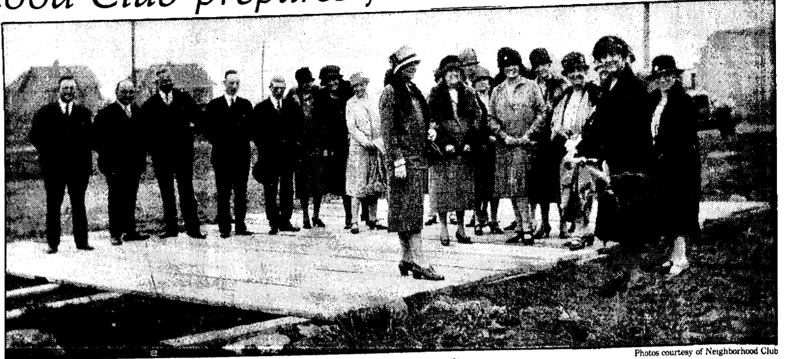
Mrs. Russell A. Alger breaks ground for the first Neighborhood Club facility.
