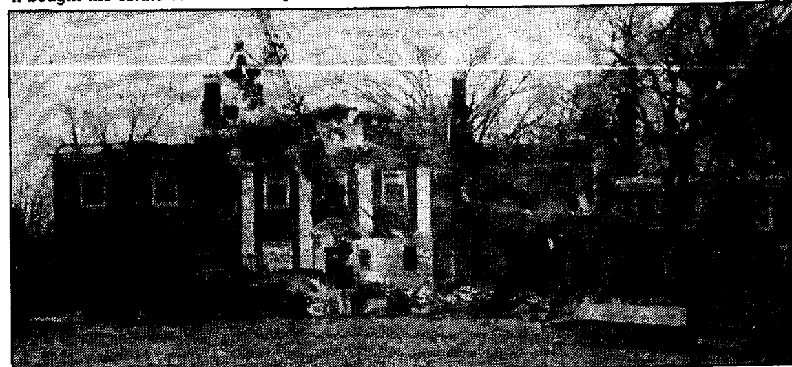
Unable to sell the Chapin House after his second divorce, Henry Ford II, he was granted permission to have the house torn down and replaced with cluster housing. Below is the pile of rubble left from what was the site of a grand Grosse Pointe mansion.
