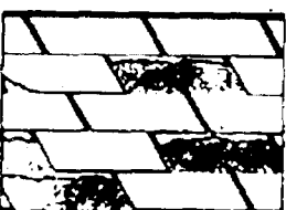
MISSING SHINGLE TABS
