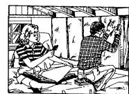
achieve that insulation level is by using high-density batts. If the sidewalls of your new living space have 2" x 6" construction, then you may want to use CertainTeed's  $5'/_2$ " thick R-21 batt. If the sidewalls are 2" x 4", CertainTeed has a  $3'/_2$ " thick R-15 batt. This batt should be used with a thin layer of exterior insulated sheathing to achieve an R-19.
