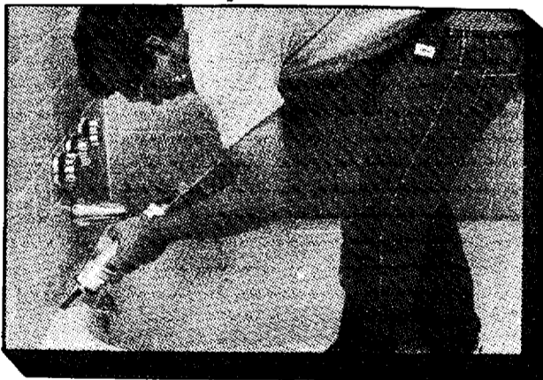
The installer uses silicone to seal the corners.
