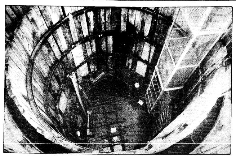
Above: The dinky track can be seen at the bottom of the 30-foot shaft; workers climb into and out of the shaft on a ladder inside the cage at right.
