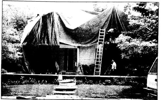
Rose Exterminators workers cover the Provencal-Weir House in preparation for the methyl bromide fumigation treatment to clear the structure of powder post beetles and carpenter ants.
