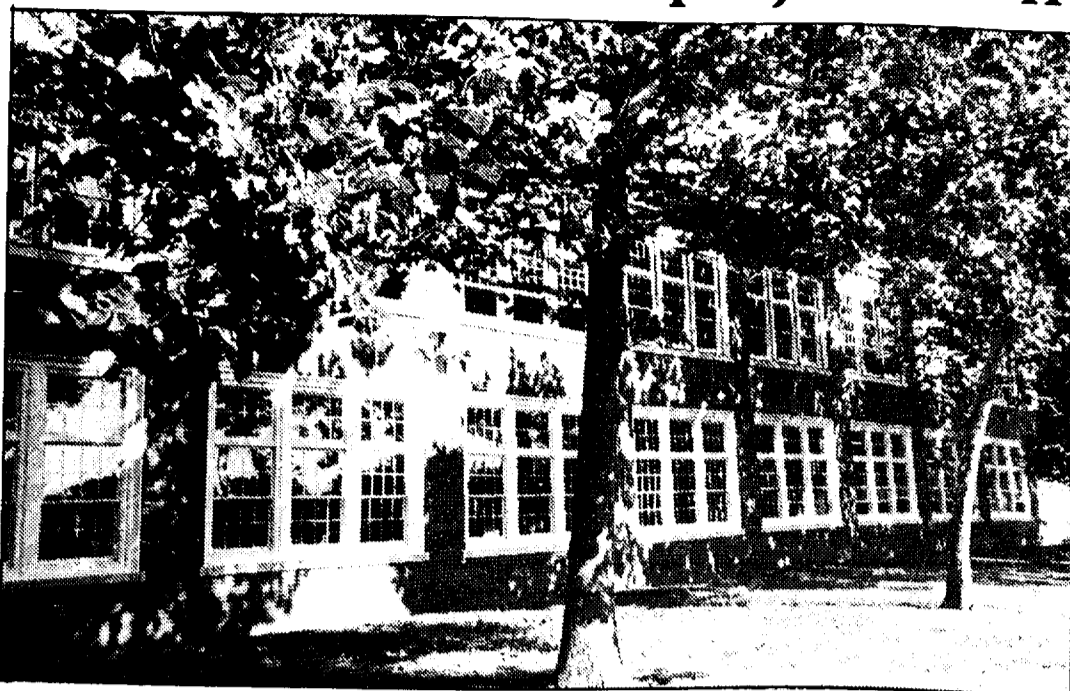
Monteith students and staff will enjoy new windows this fall, which replaced the former weather-worn, peeling windows.
