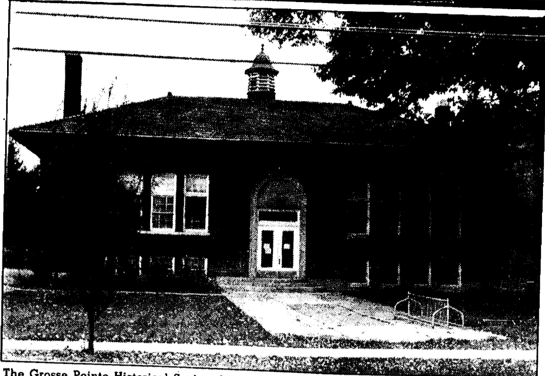
The Grosse Pointe Historical Society has sent a letter to the Village of Grosse Pointe Shores calling the guidelines the village has placed on the society's possible renovation and use of the school building too restrictive.
