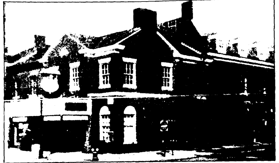
Proposed plans for the former Punch and Judy Theatre call for the exterior to remain the same while the interior is remodeled for retail shops and offices.
