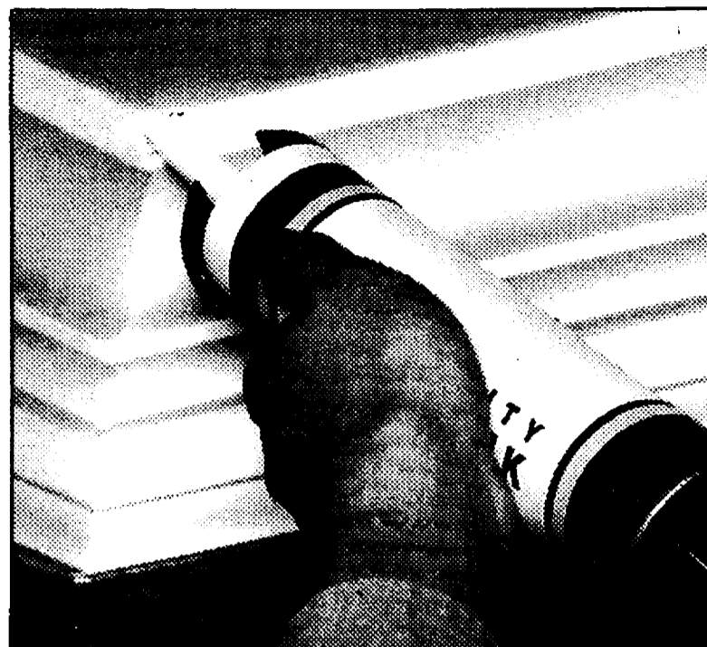
INSIDE: Caulking cracks and gaps in and around mitered joints, baseboards, chair rails or crown molding will give a room a visually pleasing, "finished" look.
