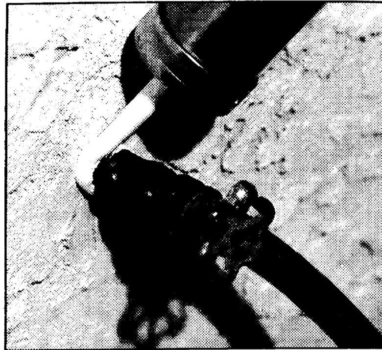
OUTSIDE: Sealing around spigots, light fixtures and other protrusions will help create a watertight and airtight seal in exterior walls.
