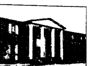
St. Clair Shores. FIRST FLOOR CONDO Sharp first floor unit with great room sizes. Freshly painted, new carpet, central air and immediate occupancy. Association exterior maintenance. Bring your fittest buyers! $64,900. #129665 (GPN-W-08RID)
