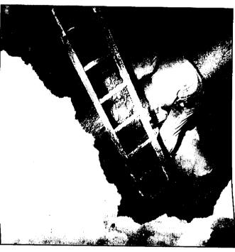
Working seven feet deep in the cross hairs of temporary utility lights, Tom Wendling, distribution foreman for the Grosse Pointe Farms water department, attaches a stainless steel metal sleeve to a broken cast iron water pipe on Meadow Lane.
