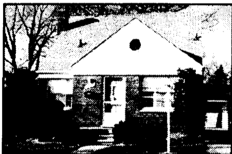
Detroit. MOVE RIGHT IN Clean and well-maintained brick bungalow. Situated in all brick neighborhood. Spacious rooms, appliances included and hardwood floors. $69,900. ☐134495 (GPN-H-51SOM)
