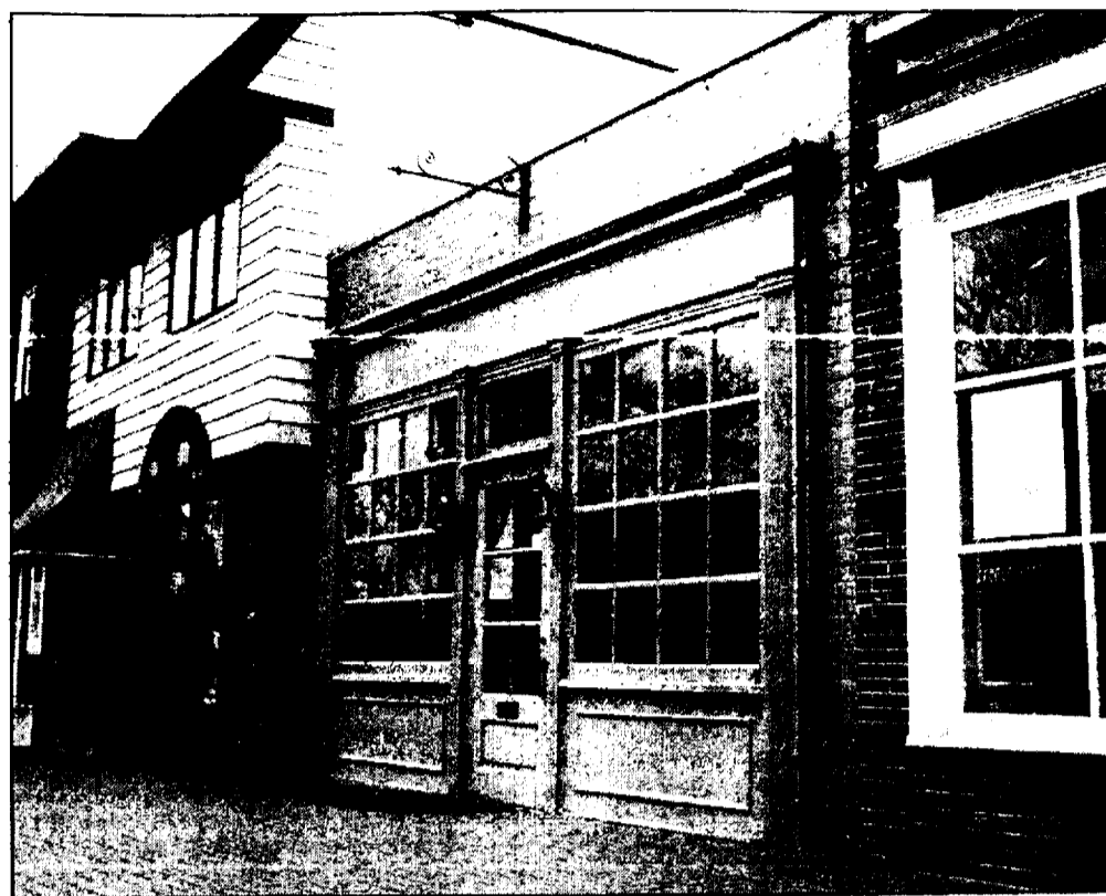
Photo by Brad Lindberg After a year delay, builder Richard Russell was granted permission Monday night by the Farms City Council to raze the former Optical Library building, center, and replace it with a new two-story retail and office building. His neighbors are the Upper Crust on the right and Something Special on the left. Russell plans to have the exterior completed by Nov. 1, barring unforeseen delays. He has yet to sign tenants for the site.
