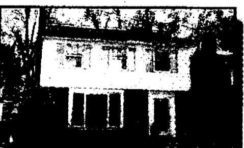
GROSSE POINTE WOODS $249,000 BEAUTIFUL, WOODS COLONIAL. Spacious living room with natural fireplace, formal dining room, new kitchen, half bath and sun room overlooking extra deep lot, on first floor. (GPN-GW-84SEV) (313) 886-4200.
