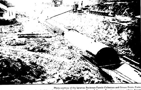
It's 1922 and the Black Marsh Ditch is being replaced by a huge sewer pipe large enough to drive a truck through. The view is of what is now Chalfonte Road near the corner of Kerby in Grosse Pointe Farms.
