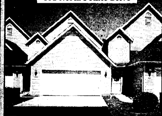
831 North Pointe Drive
