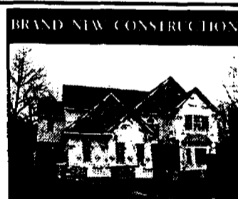
Custom built with over 4,000 sq. ft. in the Park.
