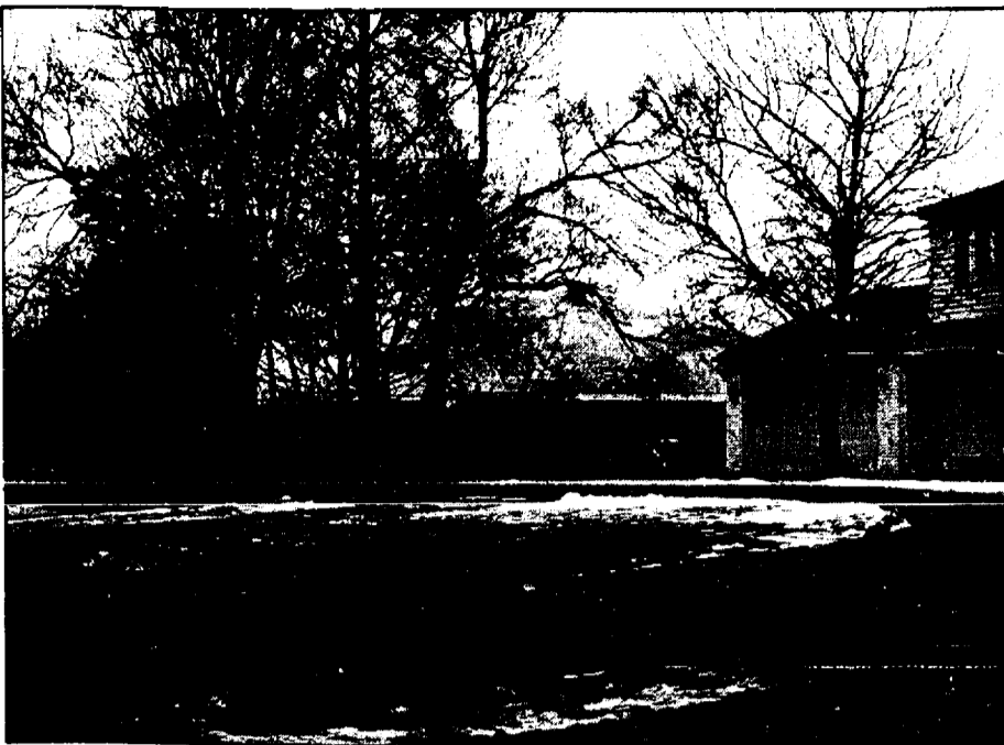
Residents of Rathbone Place and Lakeland south of Jefferson in the City of Grosse Pointe have complained that the new bathhouse currently under construction at Neff Park, shown from Rathbone Place, blocks their view of the park and lake.
