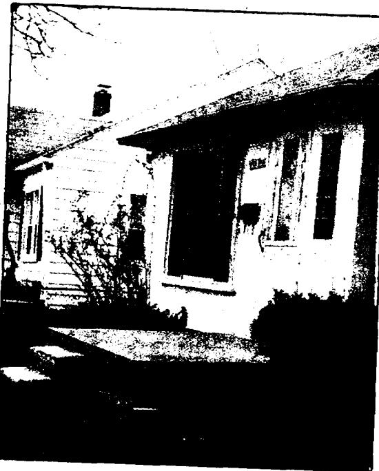
Harper Woods City Council condemned this house at 20517 Kenosha last week, sending a message to residents that it will not tolerate unsightly property. The home, which has been vacant and for sale for more than six months, is owned by a mortgage company in Dallas, Texas, which has been issued a summons.
