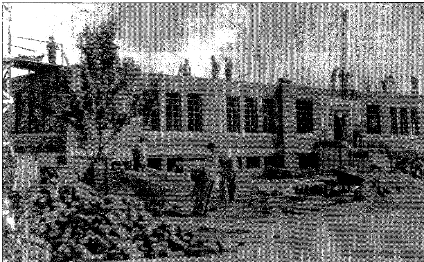
The old Neighborhood Club, 1927, under construction across the street from current club. It stood about where the tennis courts are now.
