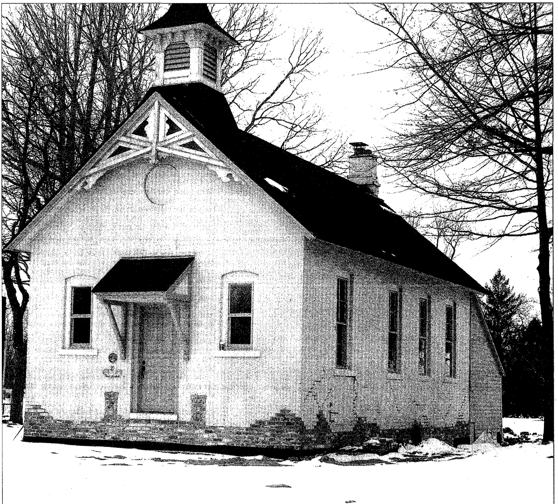
The boiler and furnace of historic Cook Schoolhouse, above, was recently noticed stolen by an unknown person or persons.
