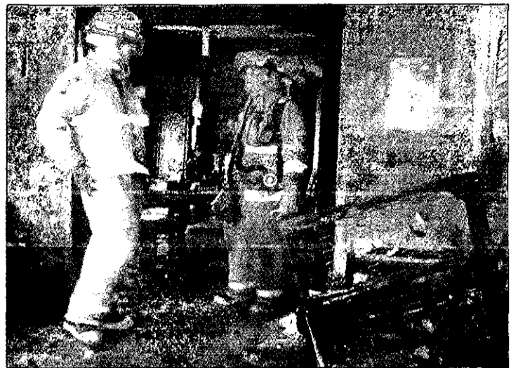
Lt. James Armbruster, right, of Grosse Pointe Park public safety surveys damage from a house fire Tuesday, May 6, fed by furniture and carpeting.
