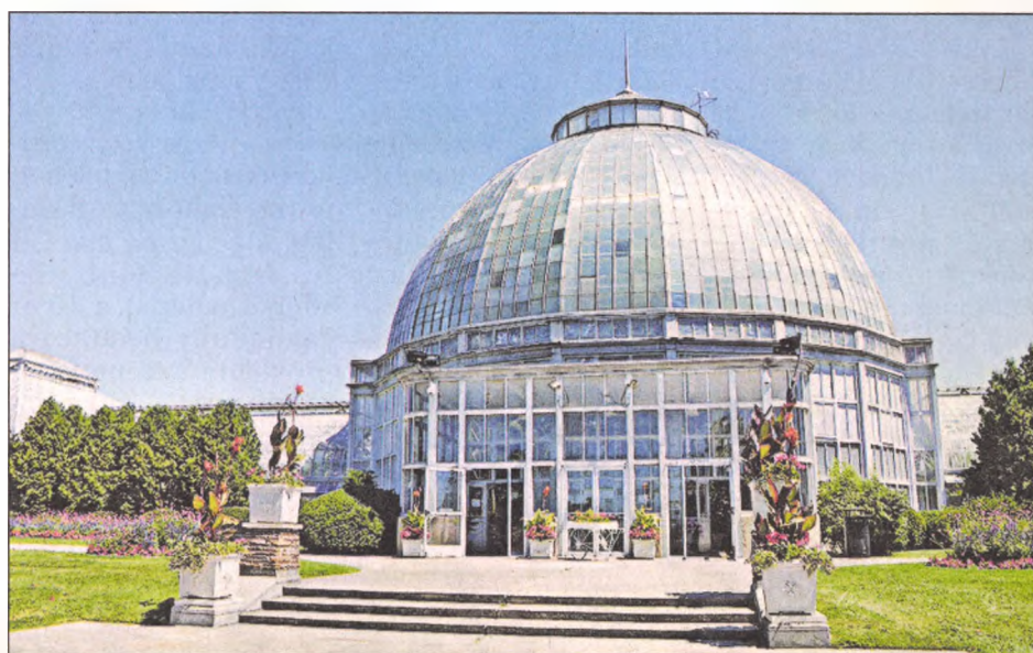
Leaking pipes and windows were replaced at the conservatory.
