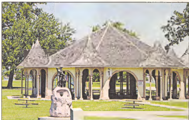
There are some picnic pavilions in need of roof repair but there are 19 shelters available.
