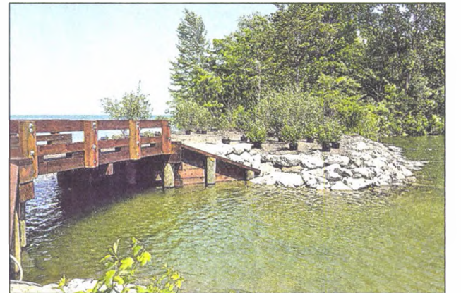
At left, the storm water project at the Ford House helps improve the ecological health of Ford Cove by directing property runoff into a newly constructed bio-swale that filters the water naturally before entering Lake St. Clair. Below, the Bird Island Bridge was built after a small portion of the peninsula was removed so water could circulate between the cove and the lake.
