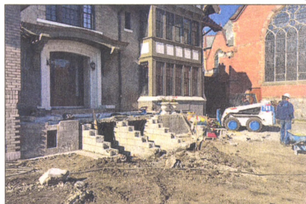
Left, exterior structural elements of the rectory needed to be rebuilt. Below, once plaster repairs were made, the ceiling was repainted.
