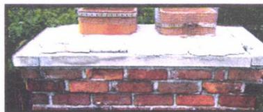
*Improperly Designed Chimney Cap*
