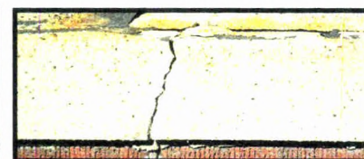
Chimney with cracked cap
