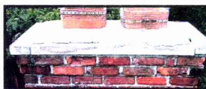
Improperly Designed Chimney Cap
