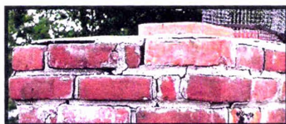
Chimney in need of brick and mortar repair with no cap
