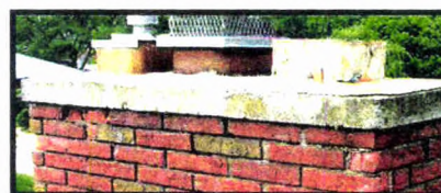
Chimney with cap damage
