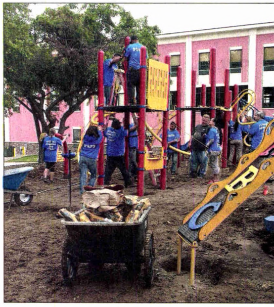
Volunteers are needed to join Grosse Pointe Rotarians and the Northeast Guidance Center Saturday, May 20, to build a community playground at the John Van Camp Community Center, 3783 Ashland, in the Mack-Ashland supportive housing neighborhood.
