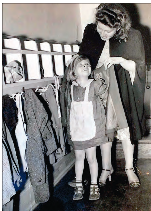
During World War II, many women went to work to backfill for men who were overseas fighting. The Neighborhood House provided daycare to support these families, including the mother and daughter pictured here in 1942.
