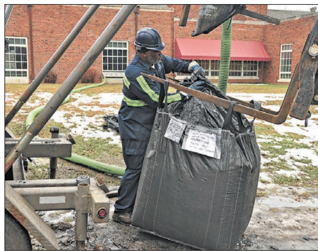
Terrence Long closes a bag of granular activated carbon and rocks vacuumed up from the floor in the vessel and puts it with the other bags to be taken to an approved landfill.
