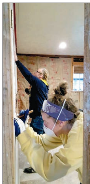
Joey Cobau and Olivia Randazzo hang drywall.
