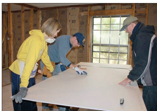
Jennifer and Mike Skalsky and Tom Cobau cut drywall for the Ray house.
