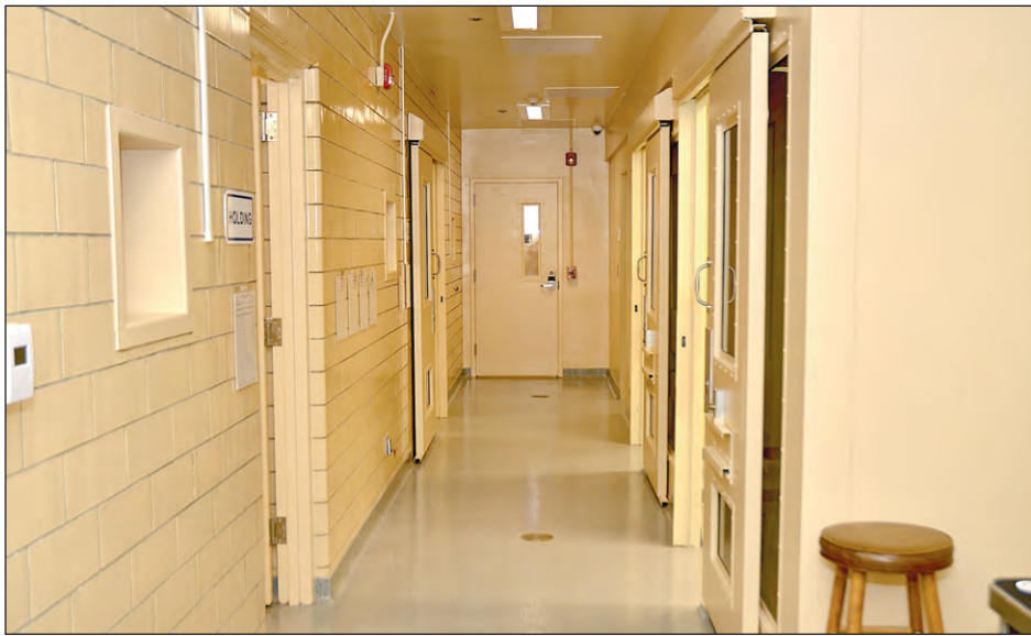
A hallway shows the new cell configuration.
