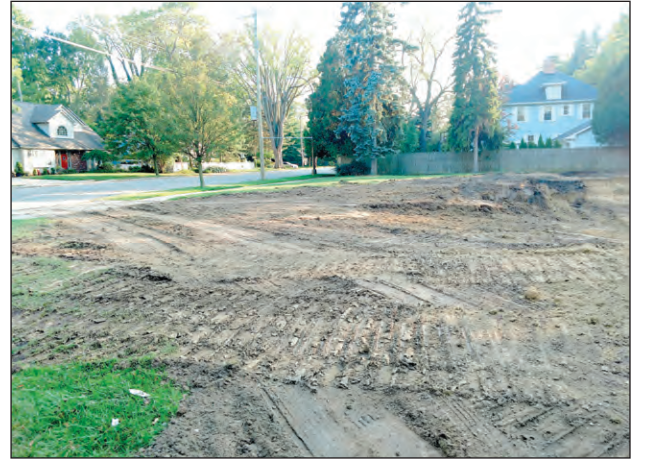
The leveled-out property after the house, shed and driveway were removed.
