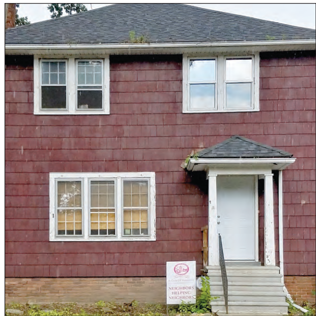
Top, the front of the house before work was done and, above, with some new windows and a new porch.
