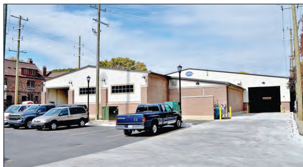
An outside view of the new DPW building.
