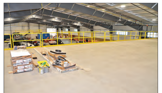
Shelving will be installed on this mezzanine, situated over the new offices.
