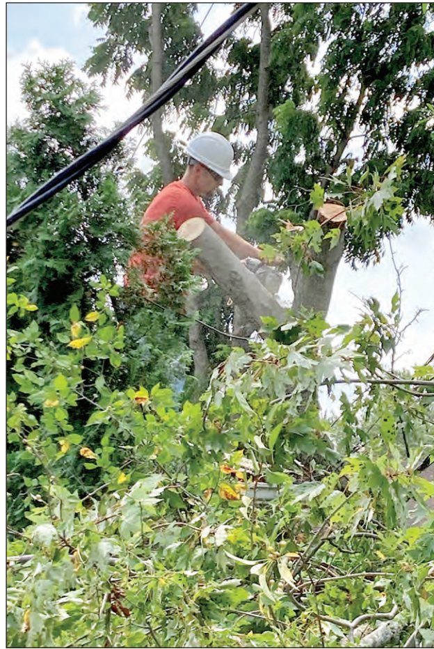
A tree contractor clears the way for DTE Energy crews to repair a power line on the rear easement between the 900 blocks of Trombley and Harcourt. High winds Monday, Aug. 9, snapped the weakened branch of a mature silver maple that fell on secondary trees and power lines.
