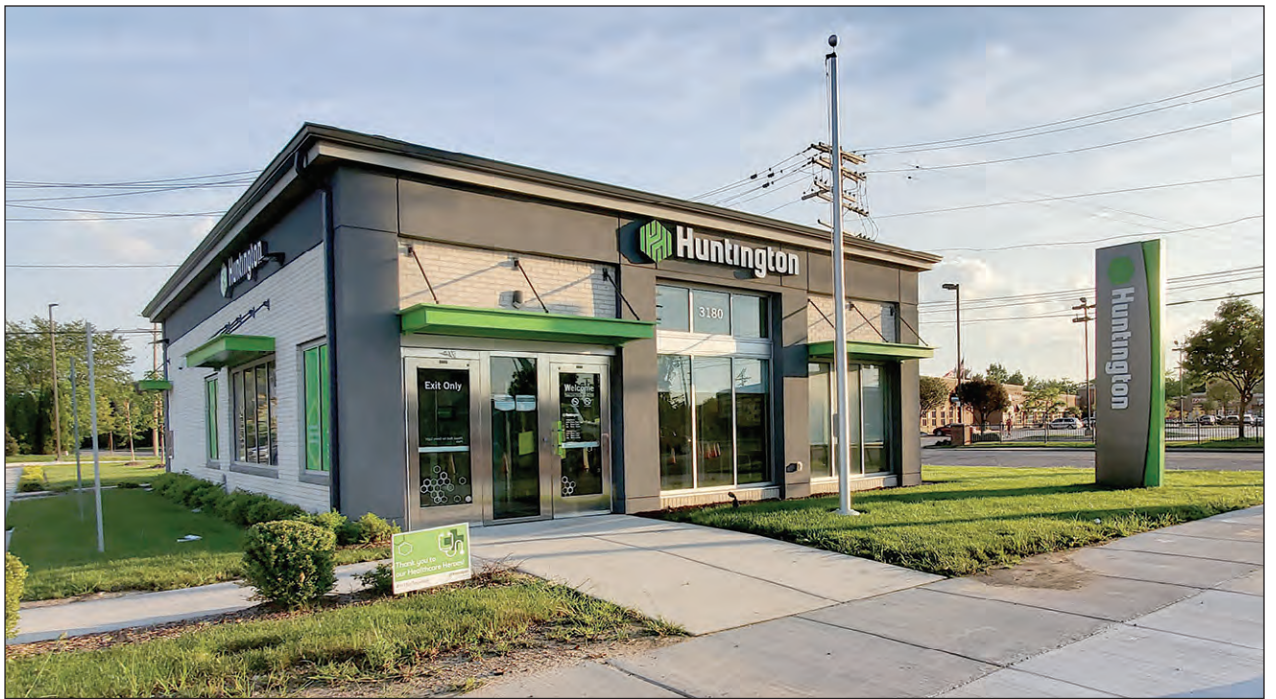
A new Huntington Bank branch has been built at Mack. And, if the council majority decides to support it, a new DPW building will be constructed next to the bank.
