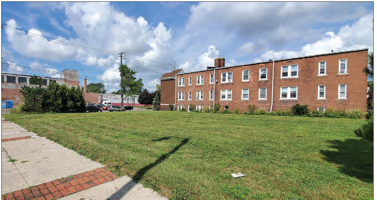
Detroit also approved the demolition of the Deck Bar (on Jefferson). This freed up additional land for the art center.
