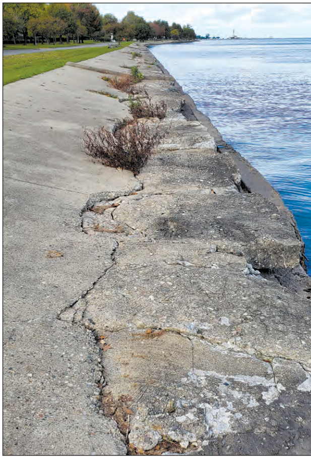
PHOTO BY RENEE LANDUYT Construction of a new seawall along the three-mile stretch of Lakeshore is estimated to cost $25 million to $30 million.
