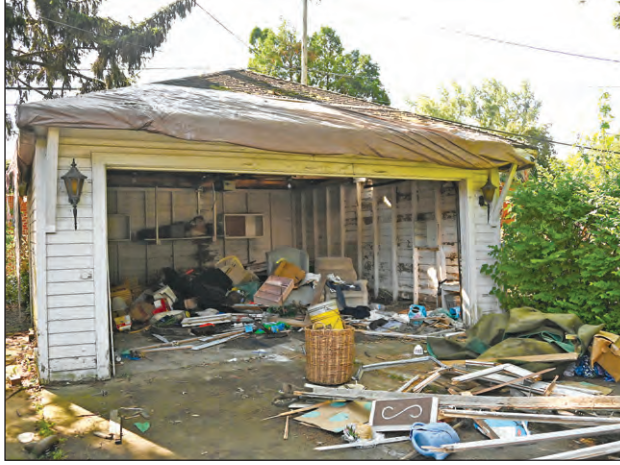
Before and after pictures of a court-ordered garage demolition on Fairway Drive in Grosse Pointe Woods Thursday, July 28. The city also tore down a garage on Severn Tuesday, July 26.
