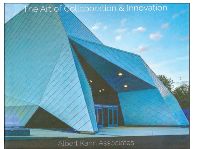
The architecture of Albert Kahn is the subject of the May 17 lecture.
